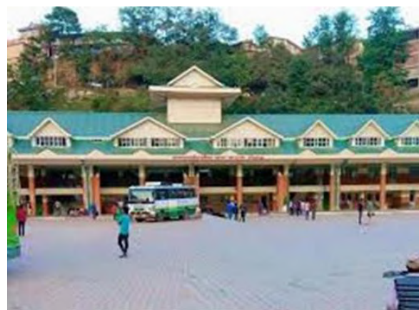
FIGURE 9 MODERN CONSTRUCTION OF BUS TERMINAL
