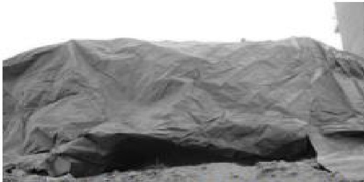
Figure 7: (Excavated Earth Covering)
