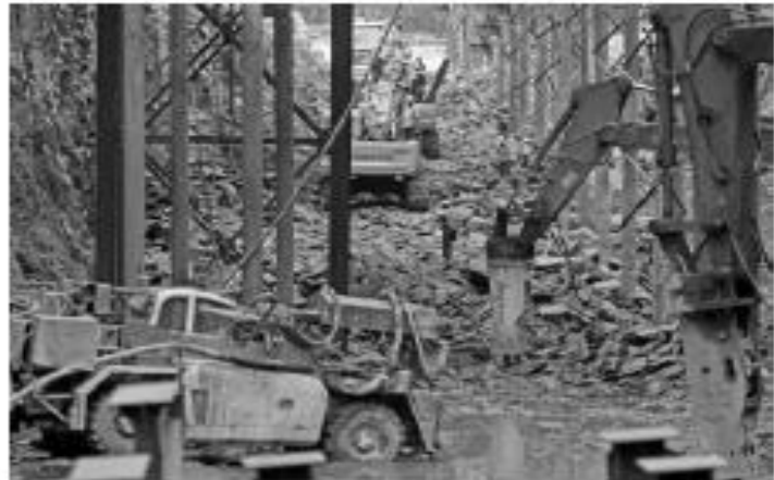
Figure 10 (Noise Pollution) (Noise & Dust Pollution by Construction Machinery)
