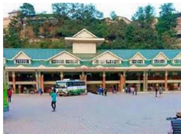
FIGURE 9 MODERN CONSTRUCTION OF BUS TERMINAL
